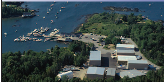
Ebenecook Harbor Southport
